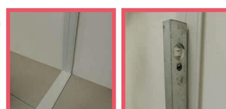
**EN:** Glue the horizontal profile to the floor. Glue the vertical profile to the wall. Check that the profile is completely vertical.
