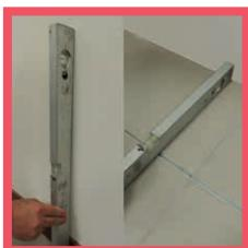
**EN:** Before to begin check that the angle between the wall and the floor is 90°.
