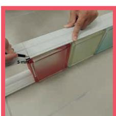
**EN:** Cut the horizontal profile. Cut the profiles 5 mm shorter than the length of glassblocks.
